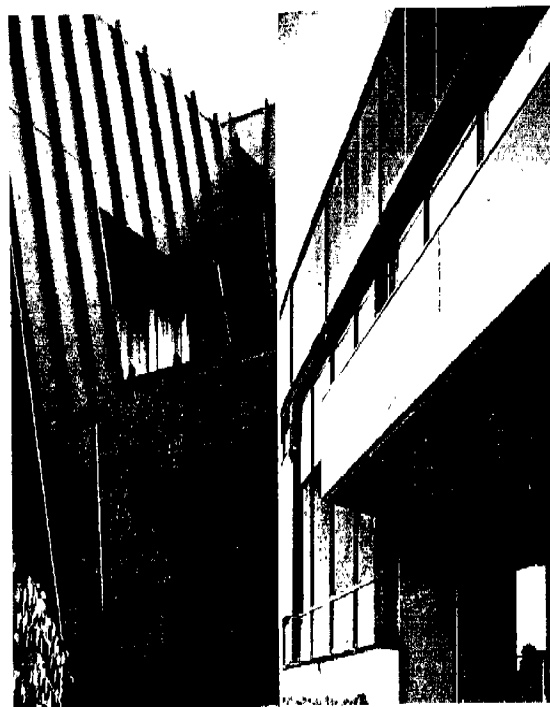
There is a great variety of applications for finished asbestos-cement sheets. Left: coloured sheets are used in the construction of a mansard roof. Right: the front and soffit ceiling of an elegant marquee are covered with coloured asbestos-cement sheets.
