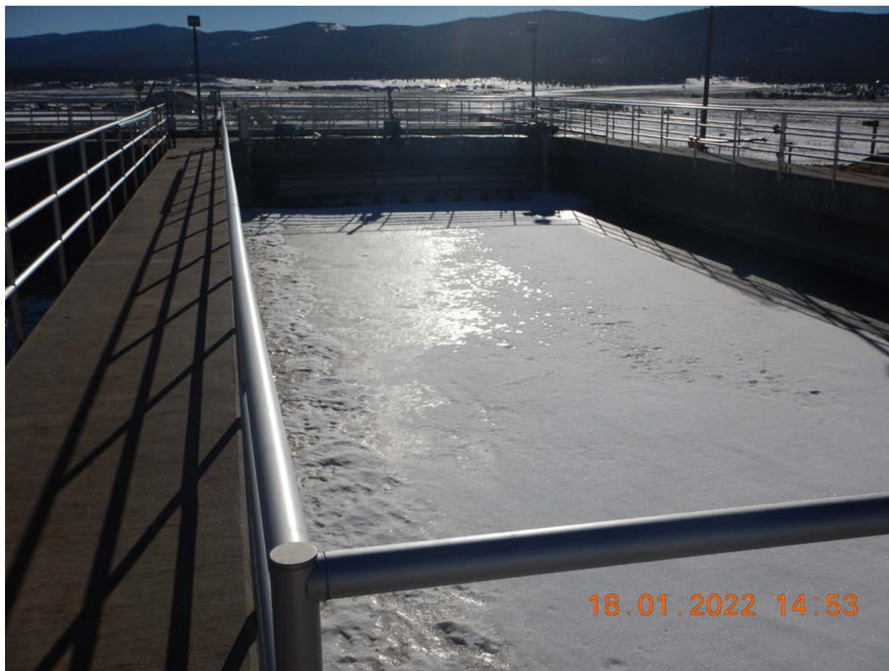
View of the approximate southside SBR currently used for treatment and storage of sludge. (DSCN 2093). Photographed by D. Esparza
