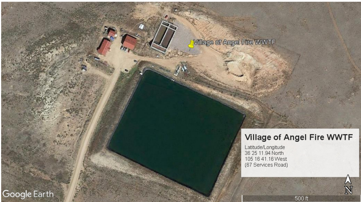
Aerial Image #1: Overall view of the Village of Angel Fire’s Wastewater Treatment Facility. Aerial from Google Earth maps.
