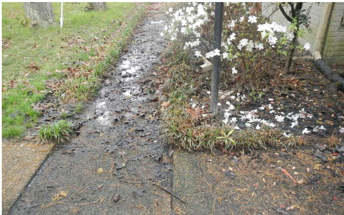
Photo 2. Raw sewage standing in the front walkway.
