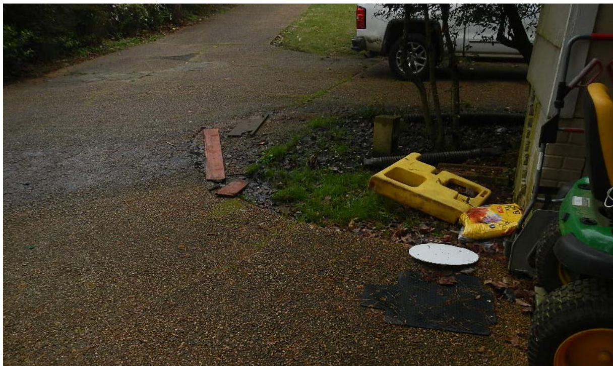
Photo 4. Sewage running across the driveway and into the yard of another resident.
