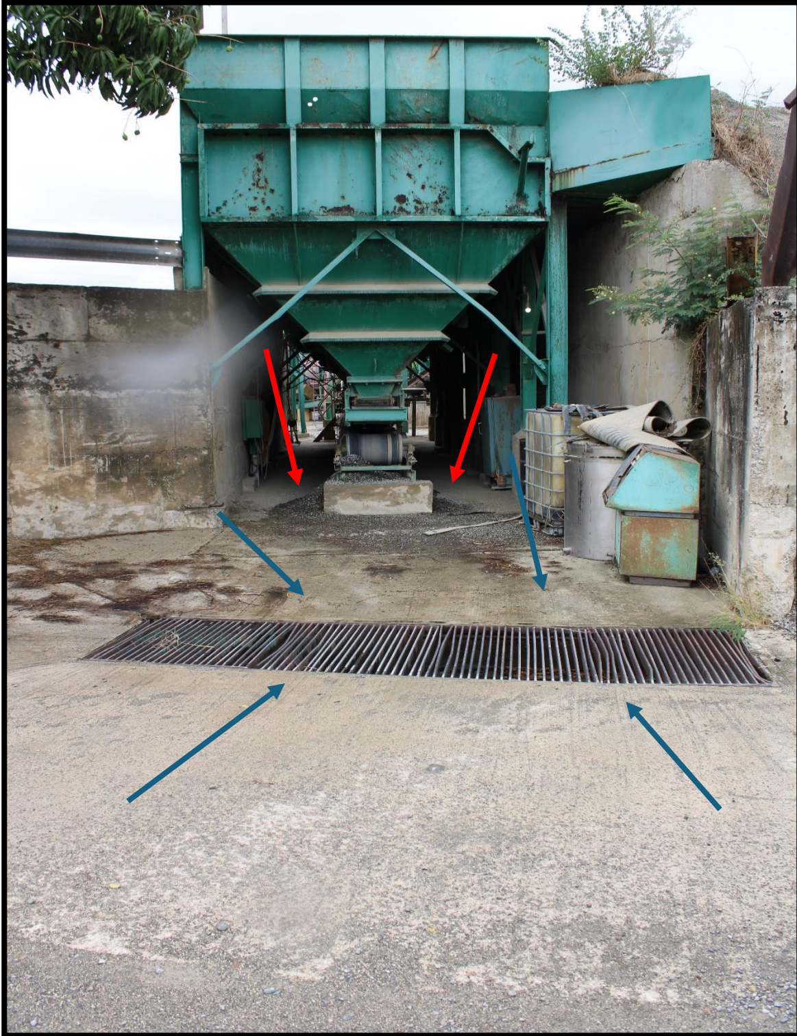
Picture 3 shows the aggregate bin feed system and a drainage grate. A tote for water storage is also visible in the picture. The holding tank was empty at the time. Unused equipment parts can also be seen. The blue arrow depicts the flow path of storm water. No inlet protection measure was observed for the storm sewer drain inlet. Also, the picture shows an aggregate spill from the bin loading machine (indicated by the red arrows).
