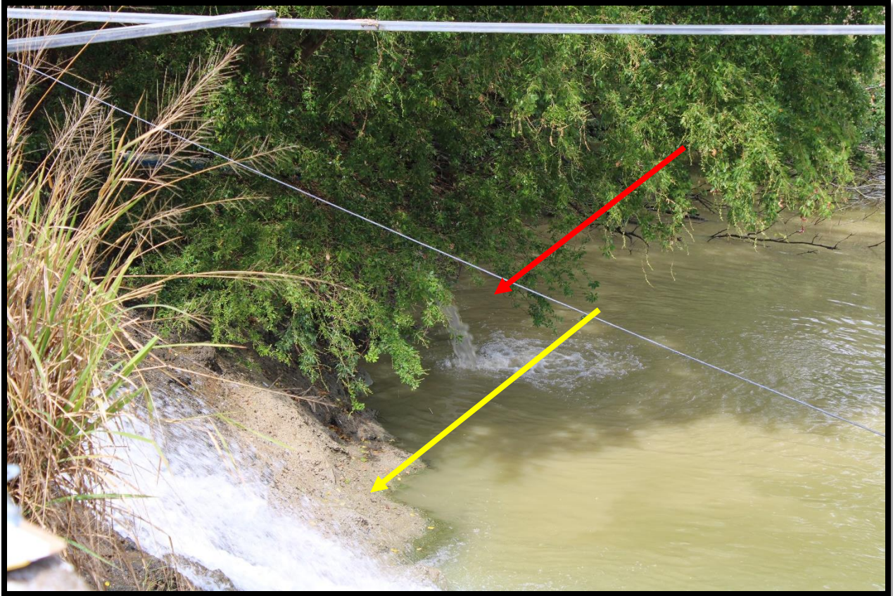
Picture 7 shows stormwater being discharged into the detention pond (indicated by the red arrow). The picture also shows water from the Inabón River being discharged into the pond (indicated by the yellow arrow).
