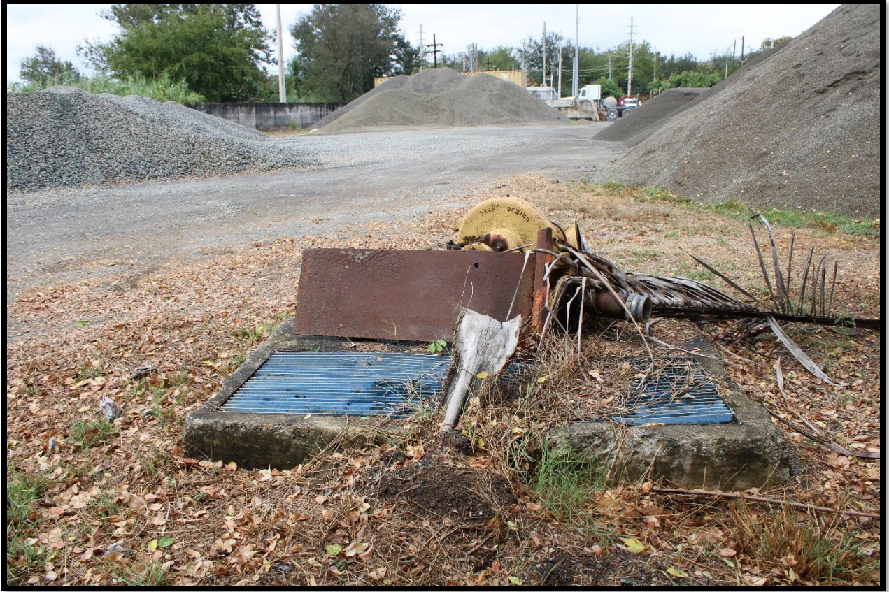
Picture 5 shows two storm sewer drain inlets next to each other without inlet protection measure and accumulated trash in the top of one of the inlet grates.
