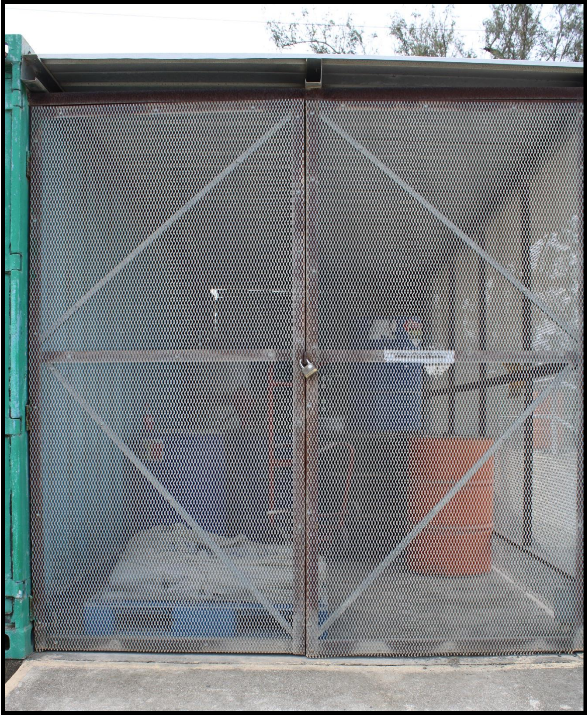
Picture 9 shows raw materials for asphalt production being stored in a covered and locked shed but lacking secondary spill containment structure.
