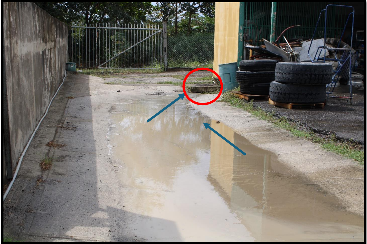
Picture 1 shows concrete swale that conveys stormwater runoff into the storm sewer drain inlet located near the mechanical shop. This drainage system collects stormwater runoff flowing from the asphalt cement processing plant. The inlet (depicted by the red circle) can be seen in the background. No inlet protection was observed. The blue arrows depict the flow path of the stormwater runoff.
