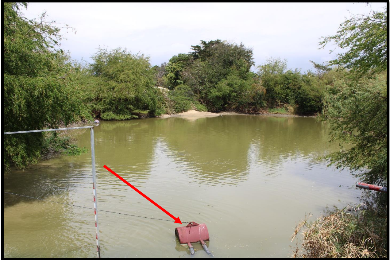
Picture 6 shows the detention pond. The picture also shows a floating device where two pipes are connected (indicated by the red arrow). There is a pump at the Inabón River that when turn-on, conveys river water into the detention pond. This system is no longer in use.
