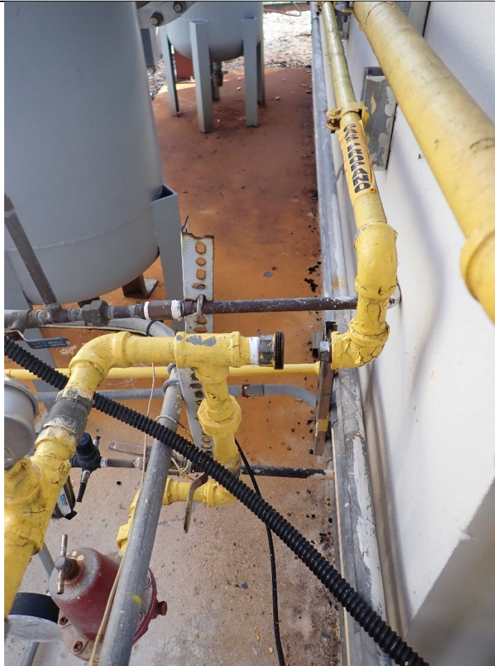
Partial view of the TO propane supply piping. The piping was cut and blinded at the time of the inspection to disconnect the TO from its propane supply.
