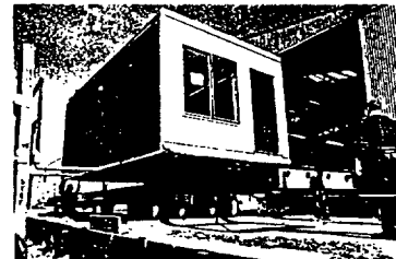
The VAC House, designed by Vencedor Development Corporation, combines the structural advantages of poured-in-place concrete with an easily assembled construction system of extruded asbestos cement components. The lightweight components are easily carried by one or two men, and may be assembled without special equipment.
