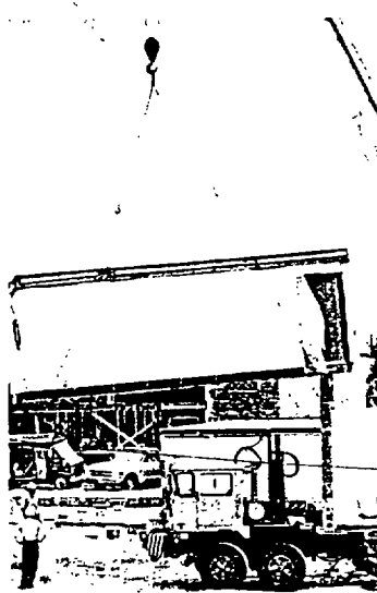
A completed modular motel room leaves the Hartford, Alabama, plant of Modular Services en route to Jacksonville, Florida, where it will become part of a new, 128-room motor inn.
