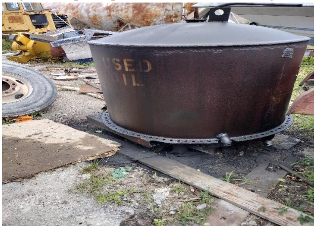
IMG 5926 -View of Facility's used-oil storage tank. The ground beneath the tank appeared very saturated from used oil spilled.
