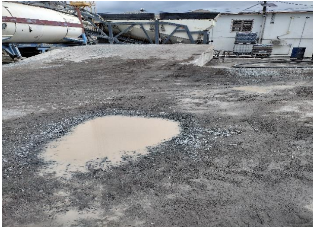
IMG 1571 -Materials build-up on and off-loading ramp of the RMCP and in path of stormwater flow.
