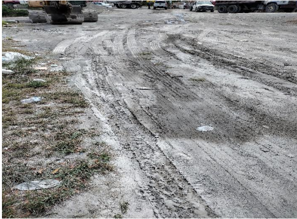
IMG 5839 -Continuation of stormwater flow path through the central section of the Facility.
