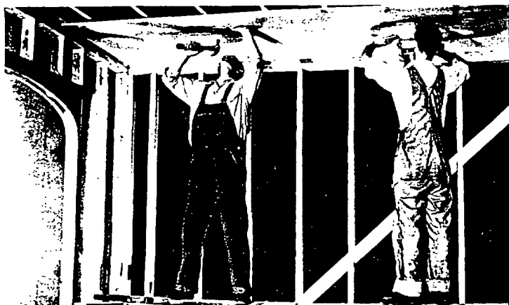
9. CEILINGS GO UP FIRST —Usually two men work on a ceiling, nailing from center of panel, towards ends and edges with nails 7" apart.
