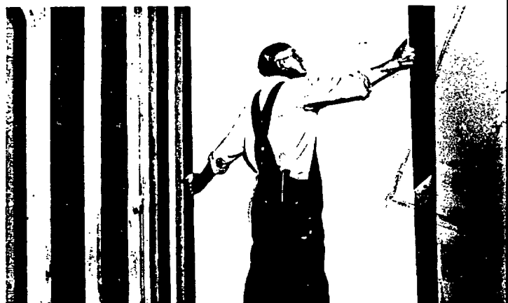
11. VERTICAL APPLICATION should be used when ceiling height is over 8'2", or where this method results in less waste or joint treatment. Boards should be accurately cut to fit, and should not be forced into place.
