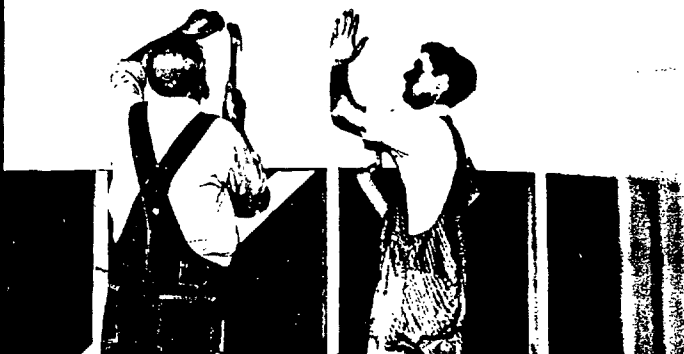
10. WHEN HORIZONTAL CONSTRUCTION is used the dry wall panel is applied first and butted against the ceiling. Over openings, end joints should be on studs. Where possible span the entire wall. End joints should be staggered. If Insulating SHEETROCK Wallboard is used, apply foil side to framing.
