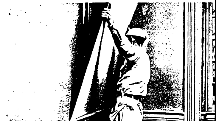
13. RESURFACING OLD WALLS AND CEILINGS —Remove all loose and poorly bonded plaster. Voids must be brought into a reasonably continuous plane with the wall surfaces by nailing SHEETROCK Wallboard in place, cut to fit and shimmed as required. Nail through SHEETROCK Wallboard and existing old surface into studs and joists with 6d cooler type nail spaced 7" on ceilings, 8" on sidewalls.
