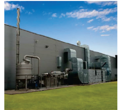
NMP recovery system from airprotech
