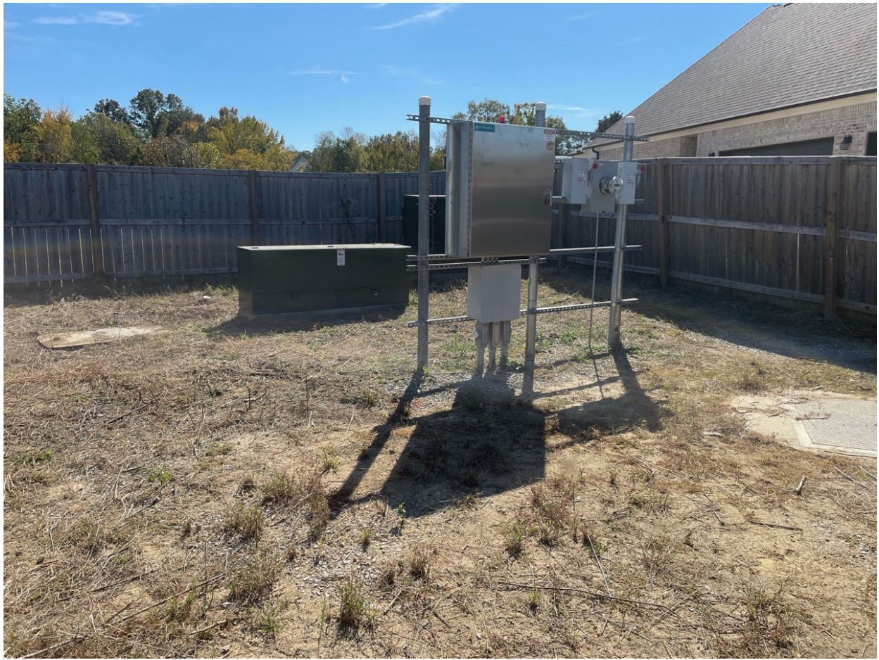
The counterweight at the North Legacy Park Lift station has been reinstalled on the check valve arm. Fencing quote obtained and PO issued for perimeter fence installation. (see above attachments).
