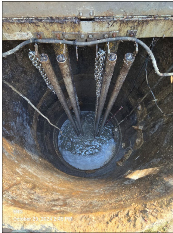
Photograph 27. East State Line lift station wet well.
