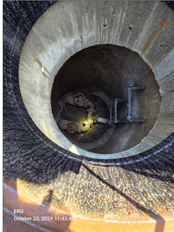
Photograph 11. Braybourne lift station valve pit.
