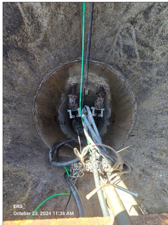
Photograph 10. Braybourne lift station wet well.
