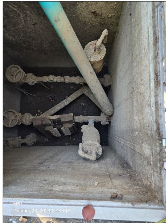
Photograph 26. East State Line lift station old valve pit.
