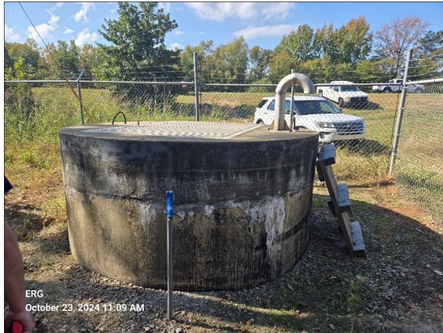
Photograph 5. Yahweh lift station valve pit.
