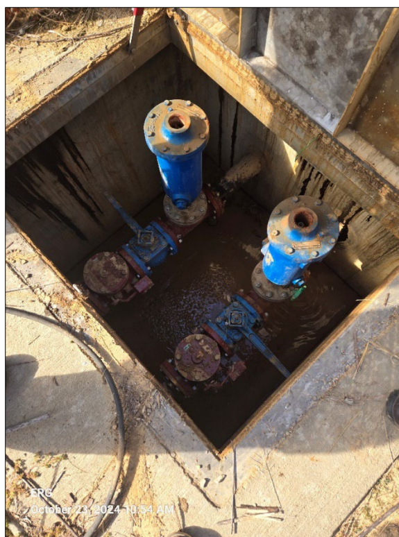
Photograph 4. McElroy Farms lift station valve pit. Note that the valve pit access is not raised.
