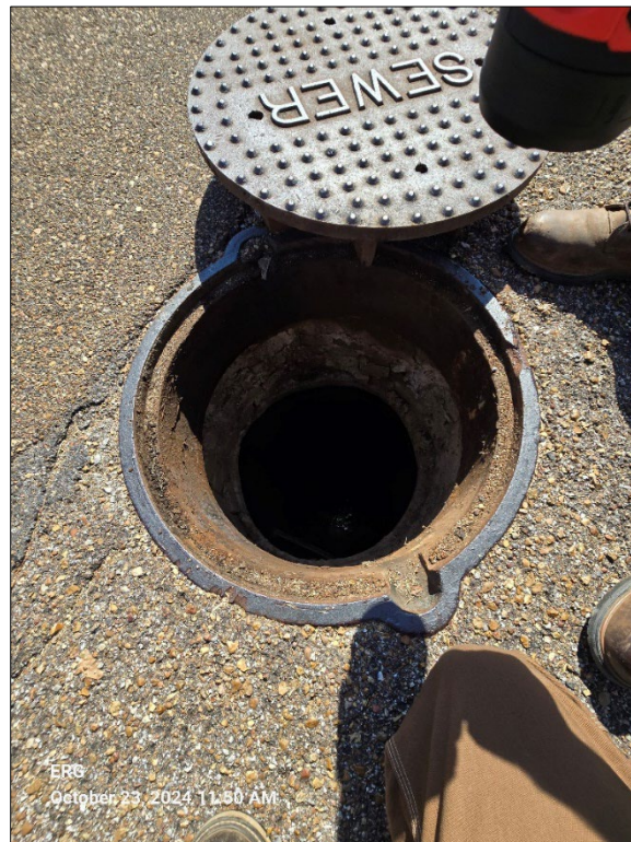
Photograph 12. Manhole at Braybourne & Sandbourne.
