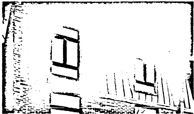
1. TERNE MANSARD ROOFS (top) were specified for unusual configuration of southwesterly of Corner Village Philadelphia, by architect Frank Weitz. Both standing and flat seams were used.
