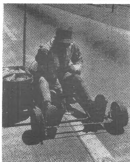
On the left a predetermined amount of adhesive is applied to specific locations on road surface with truck-mounted meter-mix and dispense equipment. On the right a button marker is hand applied on the prepared spot. The thixotropic properties of resin-grade asbestos keep adhesive viscosity constant, assuring no runoff during application.
