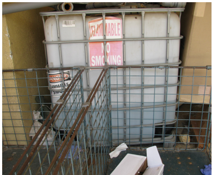
Picture 4 - GOV. JUAN F LUIS HOSPITAL, ST. CROIX- At the Hospital Backyard Area, there was one (1) 330-gallon tote containing hand sanitizer that was donated to the JFL Hospital during the COVID-19 pandemic that was in use until three (3) months ago, decommissioned and moved to this location for disposal.
