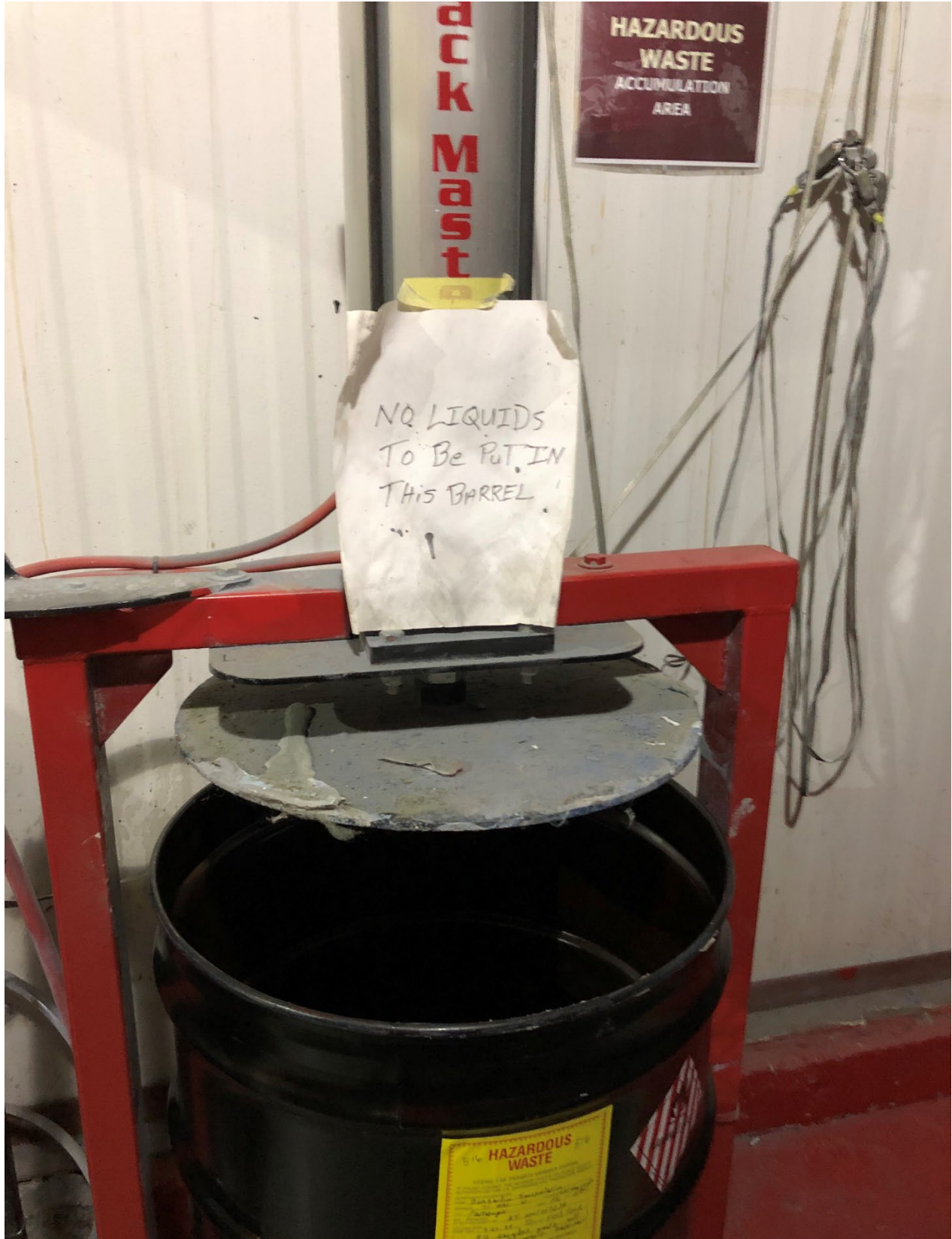
Photo #2: View of the drum of hazardous waste solids with the lid off.
