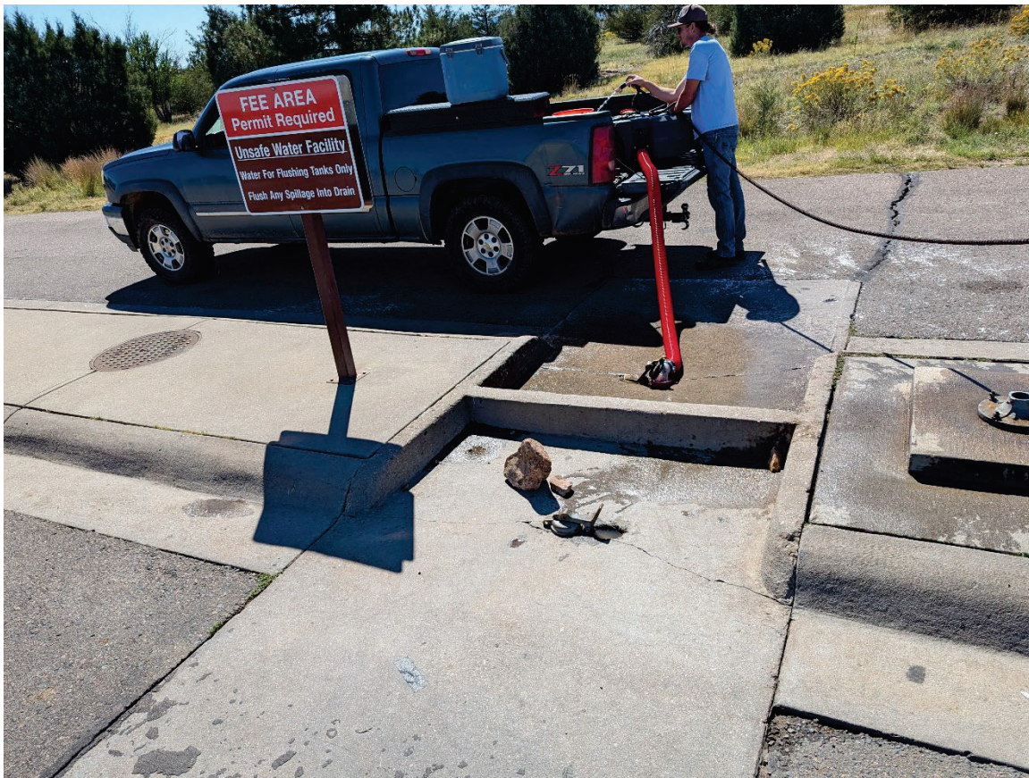
Figure 3 - Chatfield State Park - RV Dump Station
