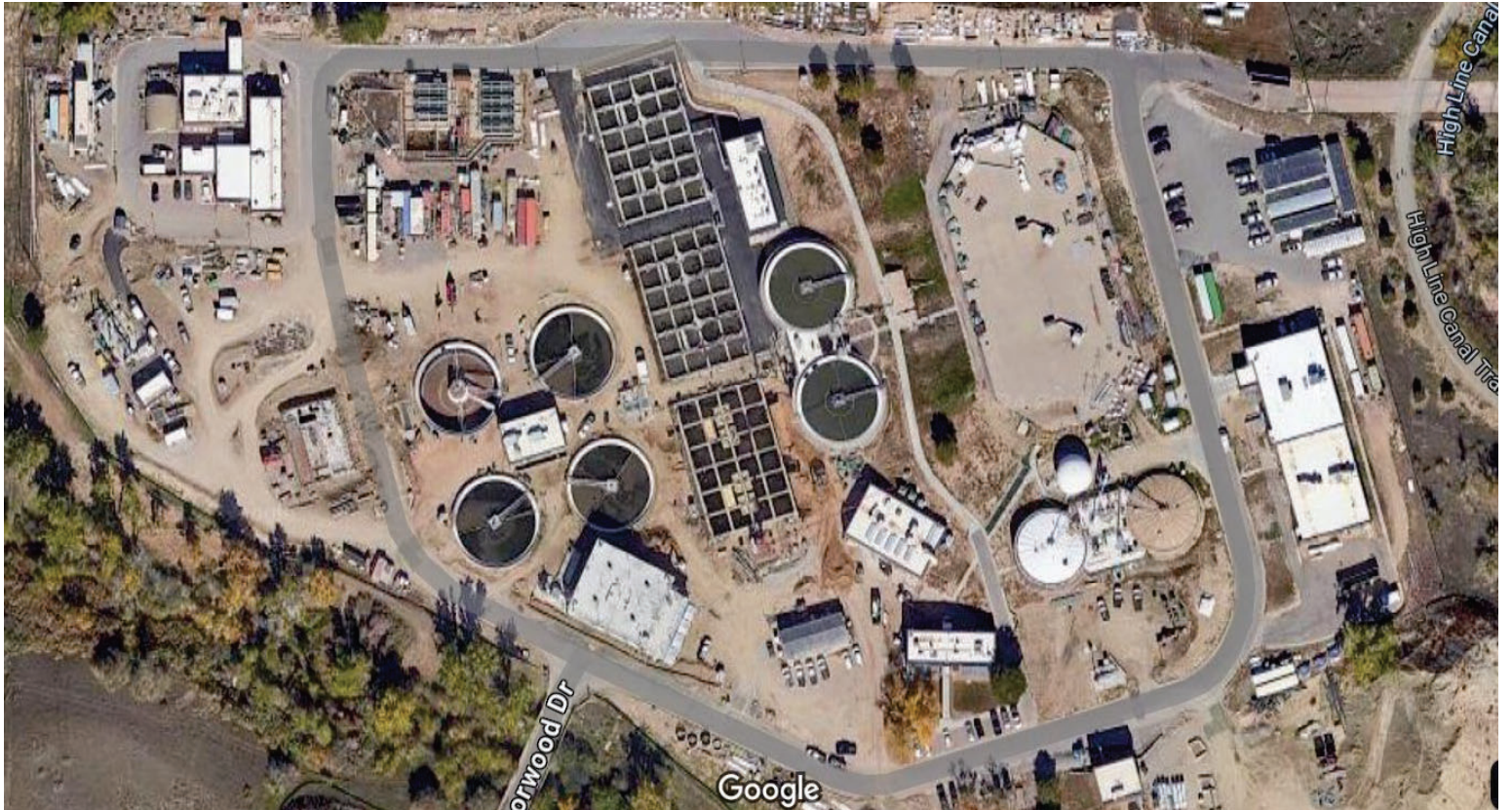
Figure 2 – Centennial Water and Sanitation District POTW – Current Google Earth View
