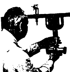
2: Next a tee is installed on the second sink by tightening the union.
