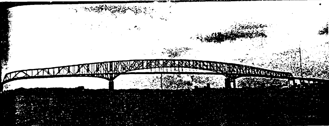
The Isaiah D. Hart Bridge, with its 1,088 foot main span is protected by four coats of lead pig- mented paints. It carries four lanes of traffic for almost a half mile between the two sections of Jacksonville on either side of the St. Johns River.
