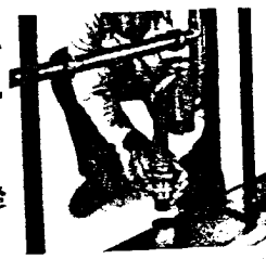
7: A trap is then added and an adapter installed to connect the assembly to an outlet.
