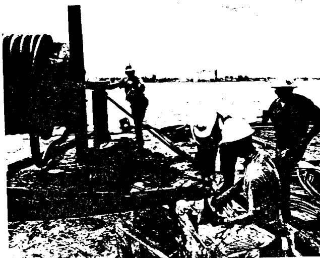
Southern Bell workmen prepare to splice a new length of lead sheathed cable into the one on the rapidly depleting reel. The three inch diameter cable is larger than the man's arm.
