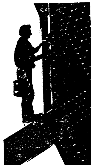
The last of the two green coats was tinted to provide a color differential.
