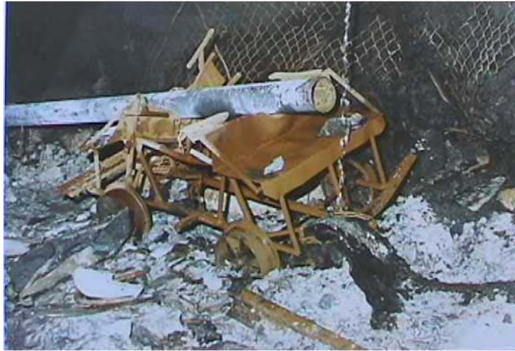
Physical damage caused by the fire
