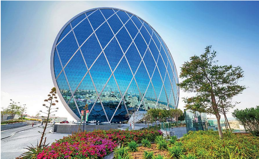
Figure 7: Al Dar headquarters, Abu Dhabi, UAE. The Al Dar headquarters building in Abu Dhabi is a 23-story structure designed by MZ Architects. It features aluminum panels coil-coated with an FEVE-based liquid coating. The steel curtain wall is also protected with an FEVE-based powder coating. The project was completed in 2010.
