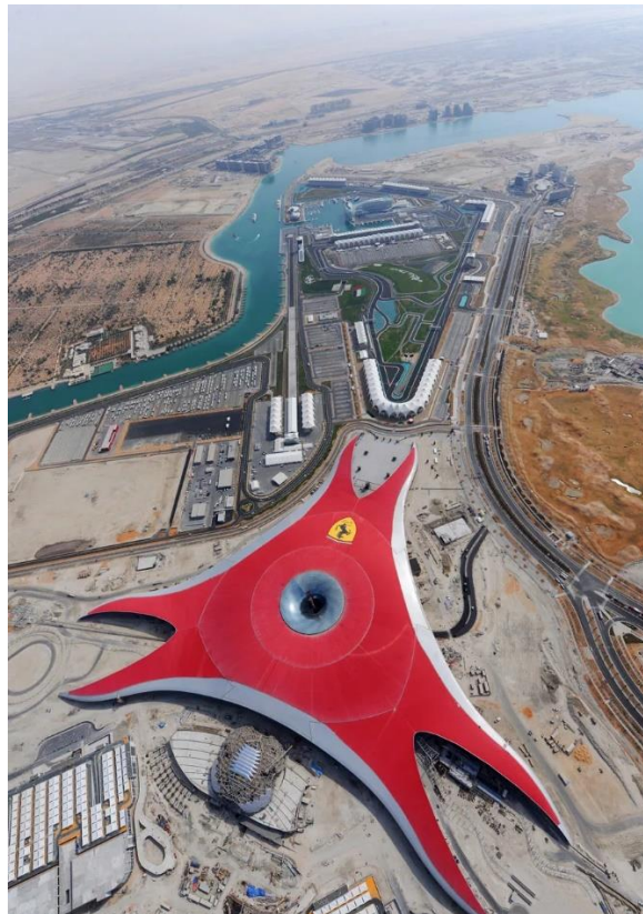
Figure 9: Ferrari World, Abu Dhabi. Developed by Aldar Properties and constructed by BESIX Group. For this extremely harsh environment (very high UV rays, located on Yas Island in Abu Dhabi) a PVDF and FEVE coating system was chosen to construct the Al roof. The project was completed in 2008.
