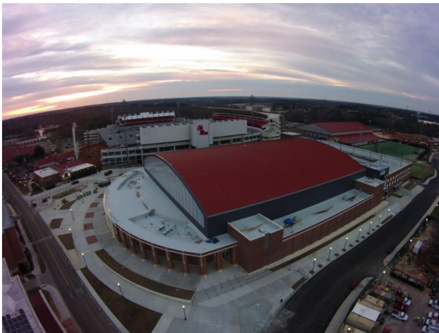
Figure 8: The Pavilion basketball arena at Ole Miss, Mississippi. The facility was designed by AECOM Technology. Chosen from an extensive list of colors, Sherwin-Williams' Fluropon 70 percent PVDF coating in Terra Cotta is a premium, high performance product that offers some of the most advanced durability and aesthetic features. The project was completed in 2016.
