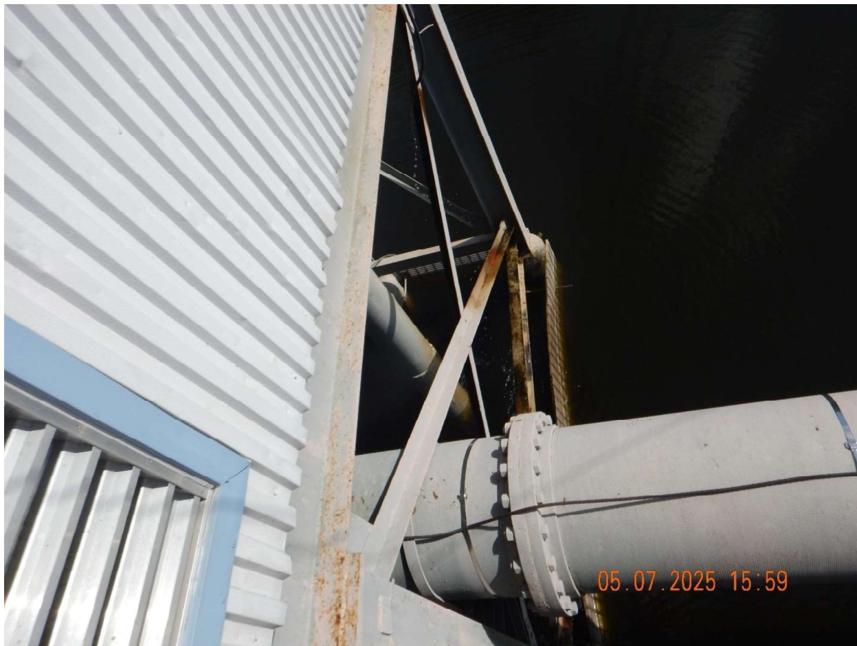
Bayou Intake View of water at intake location.
