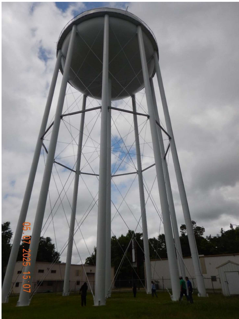
Powell Elevated Storage Tank View of Powell elevated storage tank.
