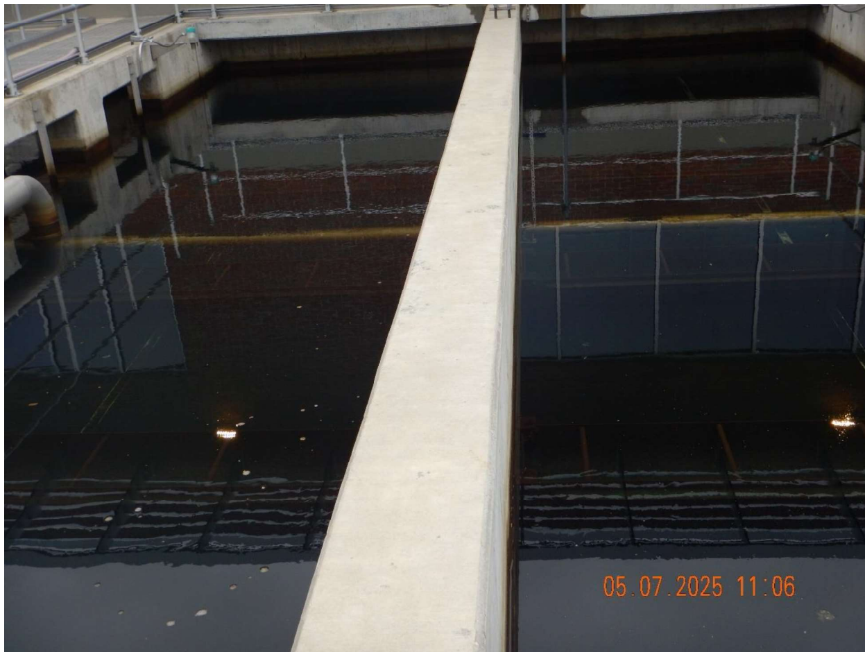
Filters View of filters.
