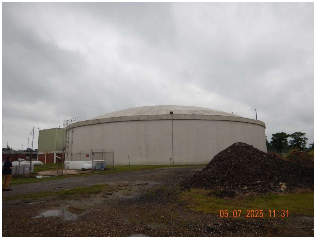
Ground Storage Tank #2 View of ground storage tank #2.
