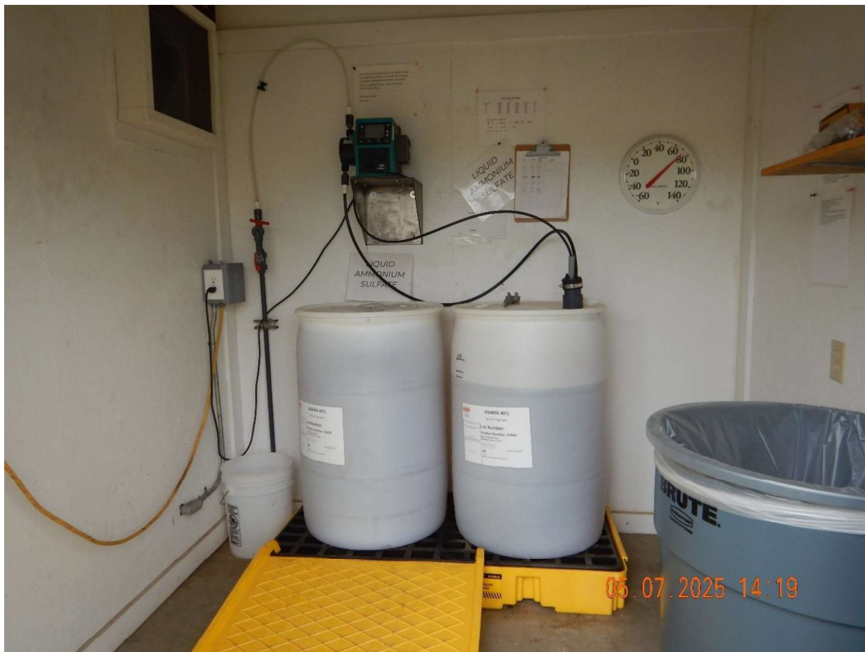
Thomas Booster Station View of aluminum sulfate tank at Thomas booster station.
