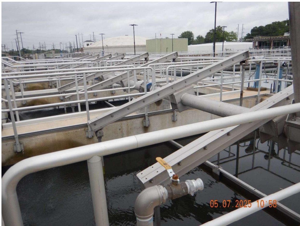
Static Mixer View of static mixers.
