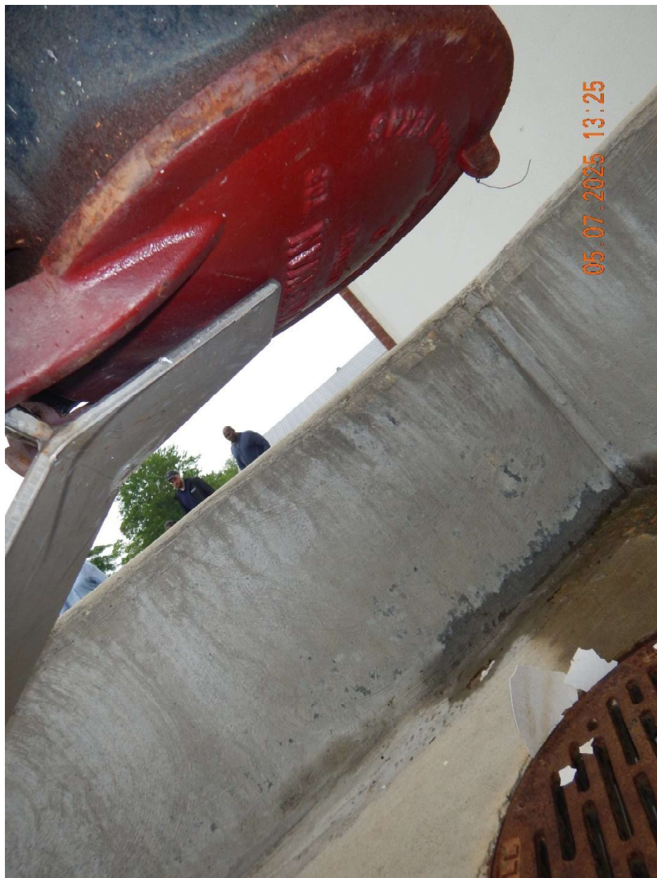
Overflow View of Chauvin tank overflow pipe with flap closed.
