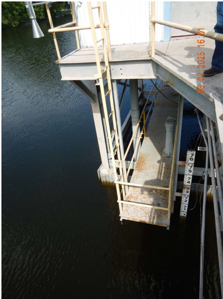
Bayou Intake View of water level at intake.
