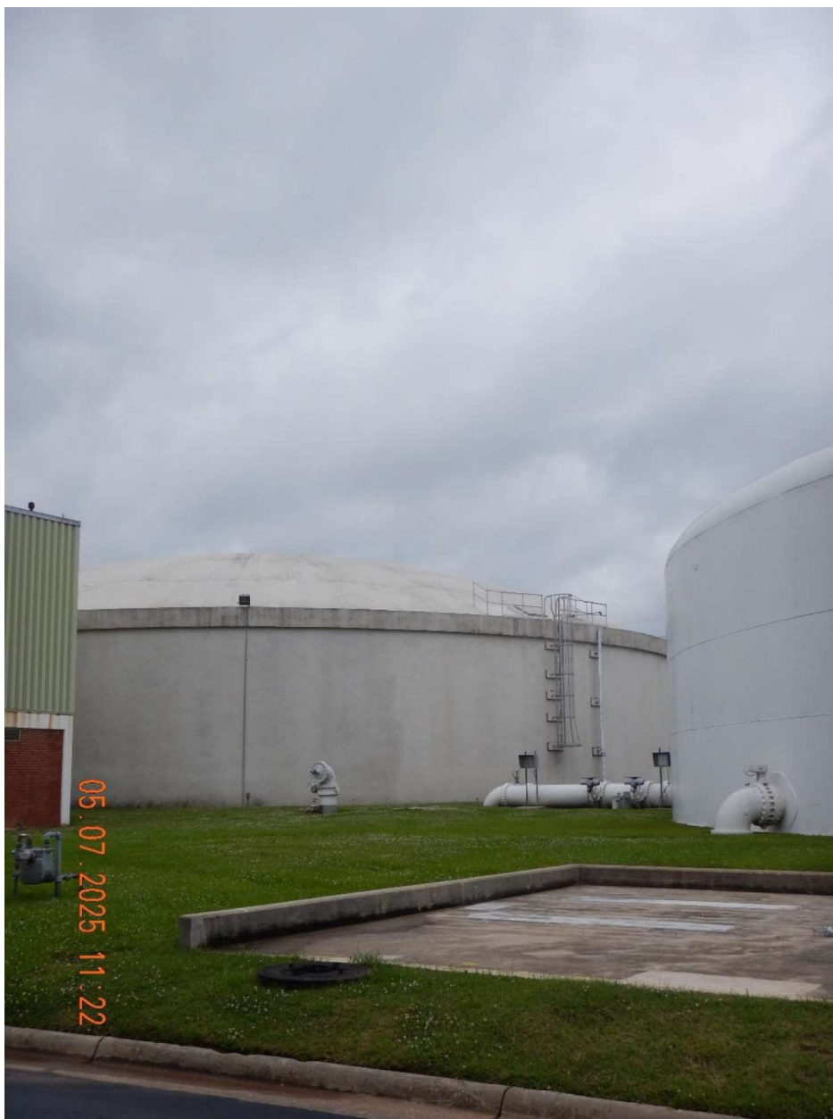
Ground Storage Tank #2 View of ground storage tank at WTP.
