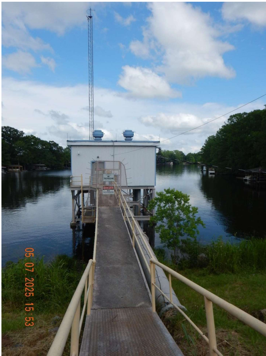
Bayou Intake View of bayou intake station.
