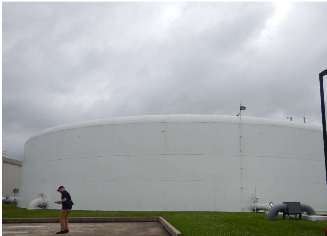
Ground Storage Tank #1 View of ground storage tank at WTP.
