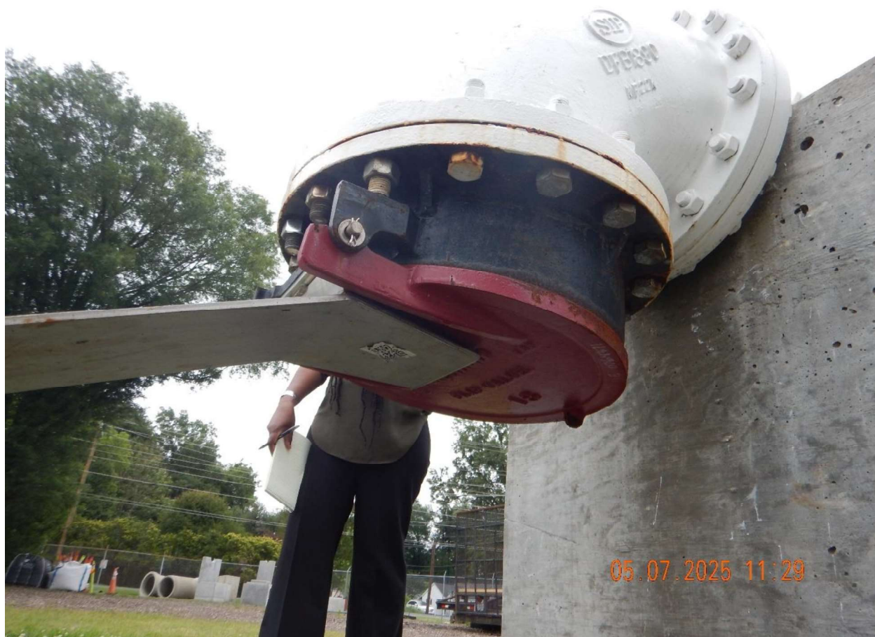
Overflow View of overflow at GST #2
