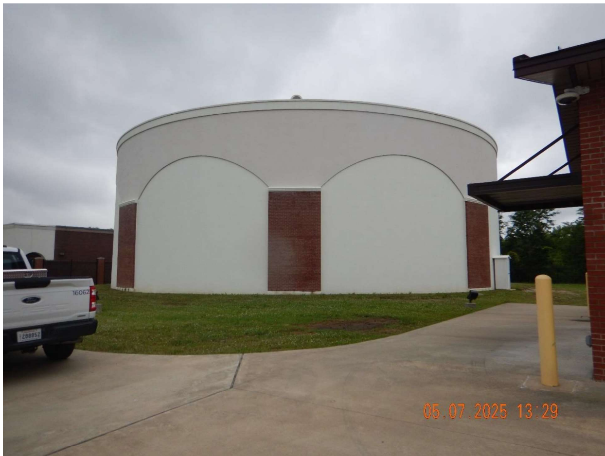
Chauvin Tank View of Chauvin Tank.
