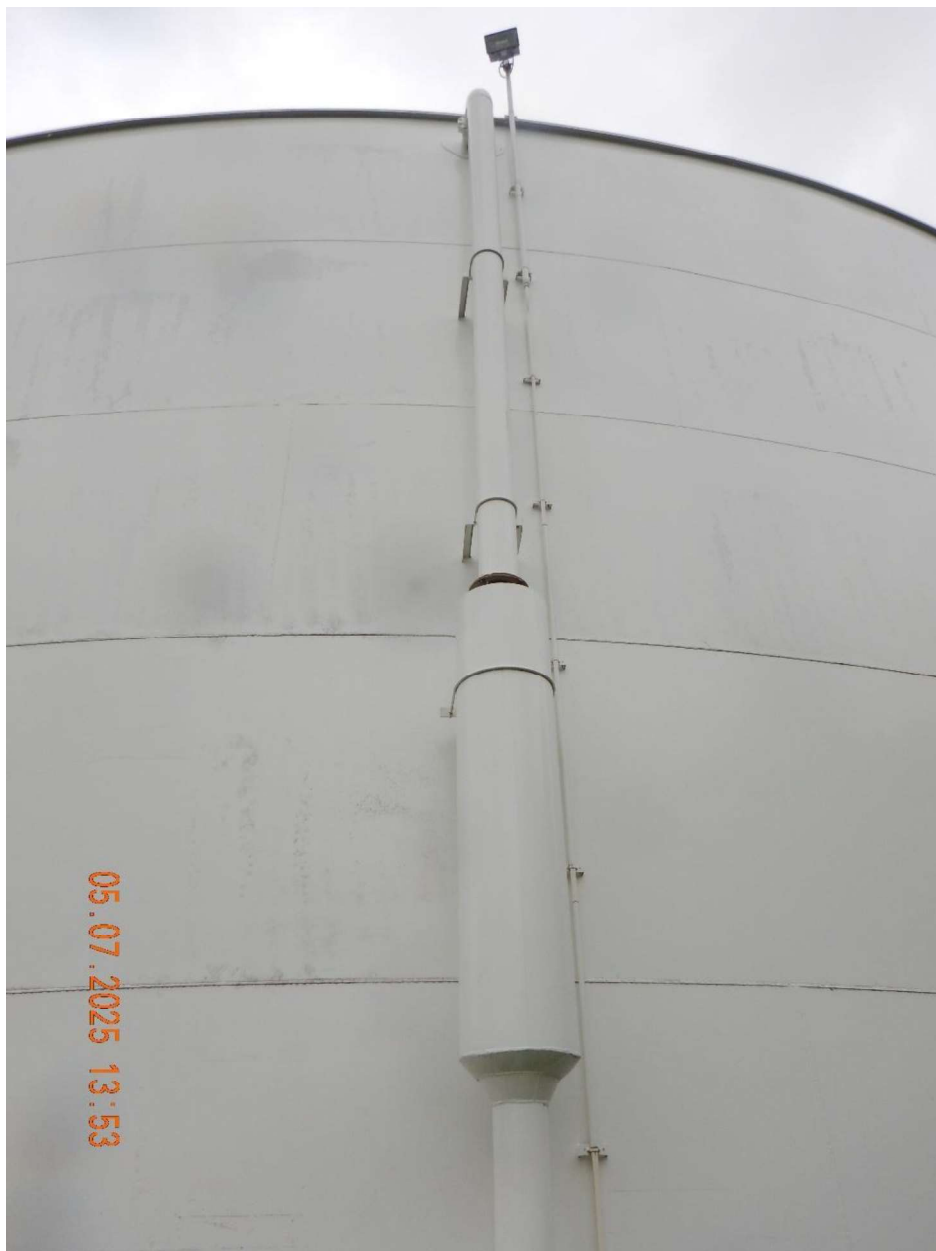
Overflow Pipe View of Ruffin overflow pipe with gap screened.
