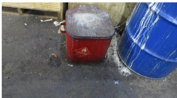
Figure 5: 11:16 AM Building 14 - Reactor Room
