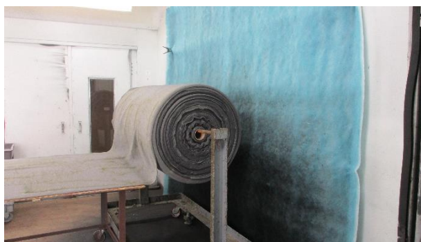
Figure 45: 2:31 PM Building 21 - Spray Booth 7
