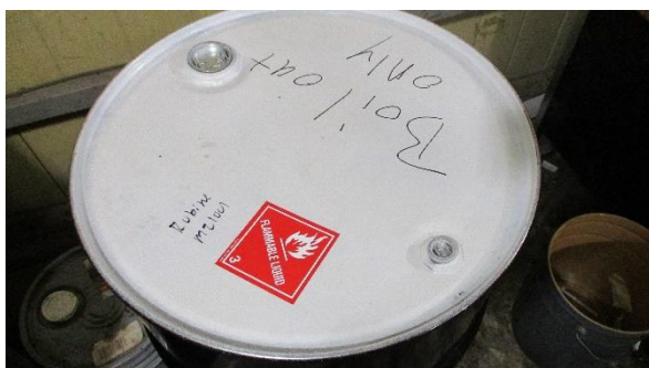
Figure 6: 11:26 AM Building 14 - Reactor Room
