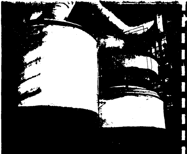
Converters used in manufacture of sulfuric acid at Everett, Mass. plant.
