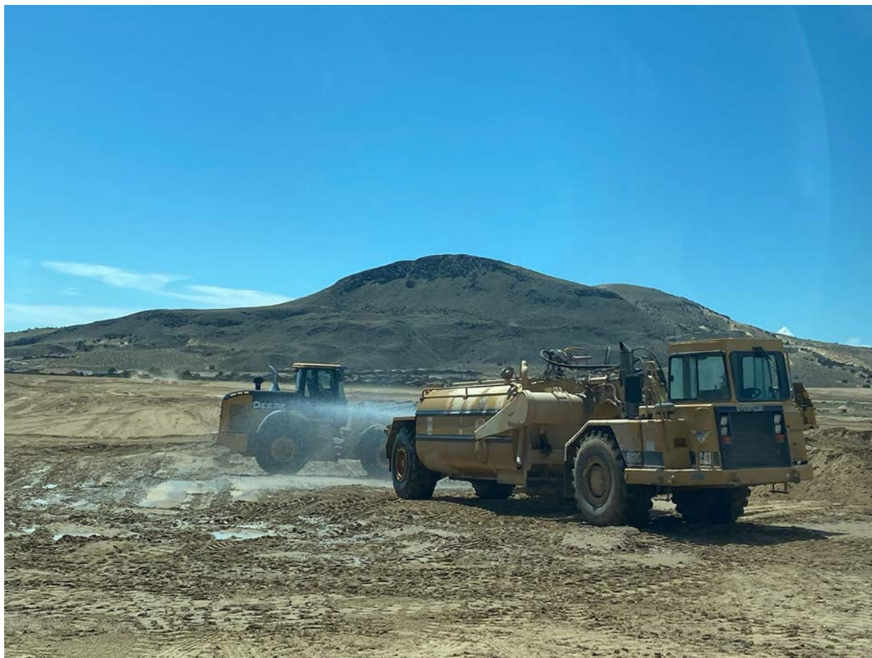
Greater Kudu/Facebook Project Antelope Phase II dust suppression efforts utilizing water application. Photograph provided by Greater Kudu/Facebook.
