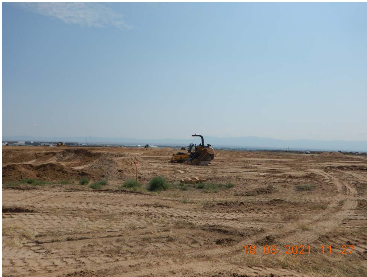
View looking approximately East of earthwork inside the Facebook facility. August 18, 2021 (DSCN1957).
