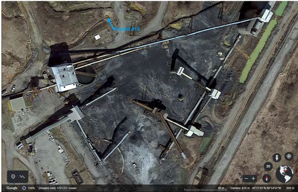
Image 3. Aerial image of Outfall 010 near the conveyor belt. White square indicative of the cover built to prevent dust from conveyor belt from blowing into the sand filters.
