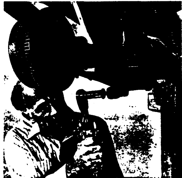
Fig. 29 — Disconnect the shock absorbers.
