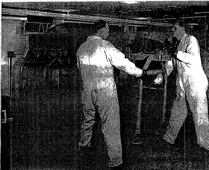
At Oak Ridge, portable tunnels with 3 inch lead walls are used to shield radioactive samples drawn from the uranium-graphite chain reactor. (Union Carbide & Carbon photo.)
