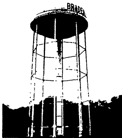
Jacking equipment attached to the support structure's legs allowed Bradenton's new water storage tank to be raised an additional 3.7 m (12 ft).
