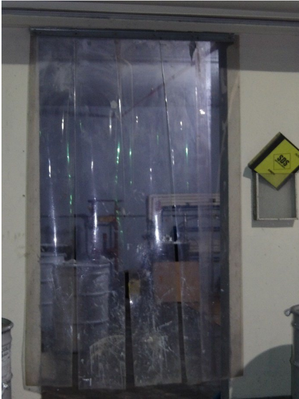
Photograph One (1): Outside Overview of the Paint Room SAA
