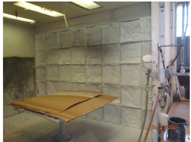
Picture 50 – Spray Booth paint filters
