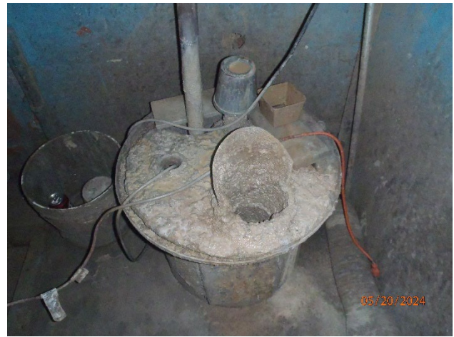
Picture 4 – Sanding Staining WW sump and used cloths
