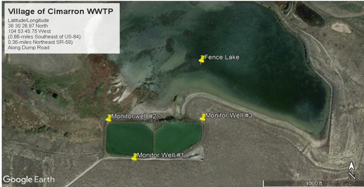
Aerial Image #1: Overall view of the Village of Cimarron's Wastewater Treatment Plant. Aerial from Google Earth maps
