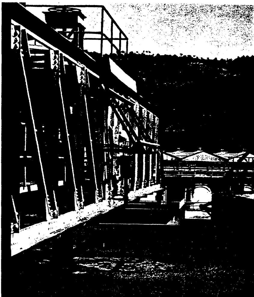
Cyanamid's Superfloc* RM30 red mud flocculant is used in this washer at Alcan Jamaica's plant near Mandeville, Jamaica. The flocculant speeds up the settling process in which alumina is separated from bauxite ore residue, one of the early steps in the manufacture of aluminum.
