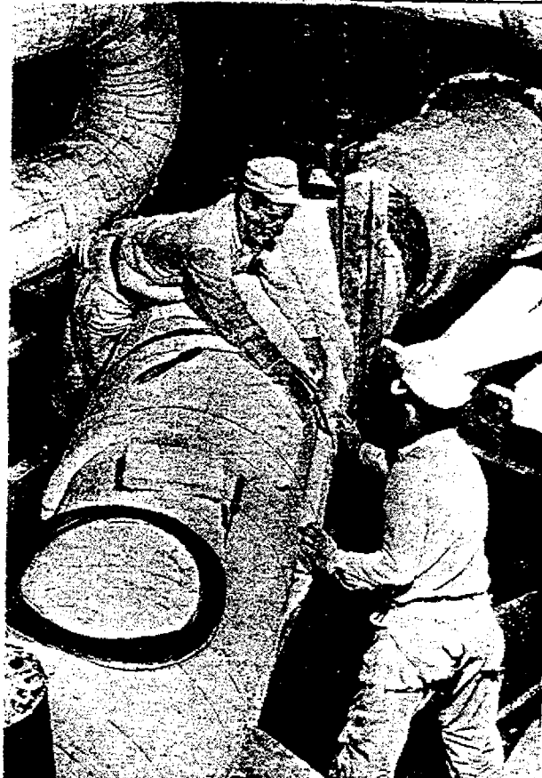
STEAM MAINS being covered with high-temperature insulation
