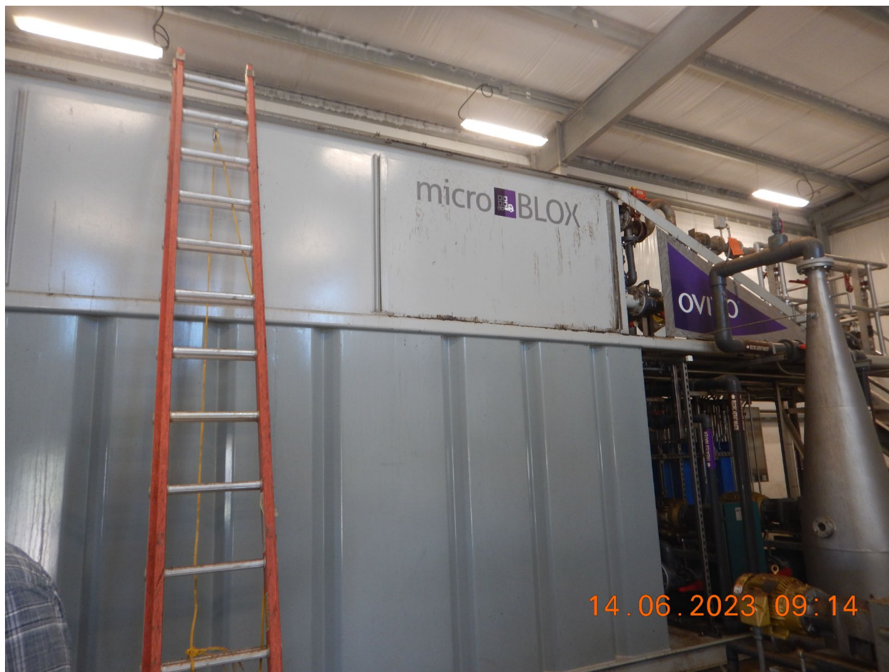
View of the Ovivo• microBLOX™ membrane bioreactor (MBR). (DSCN2570) Photographed by D. Esparza
