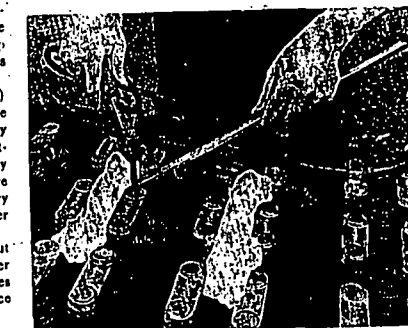
5 Burn joints with a carbon rod connected to three battery cells. Apply fresh lead so it flows into melted puddle
