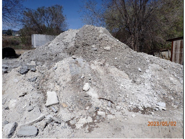
Photo #:10 Description: Facing west, photo of pile of debris from truck washout.
