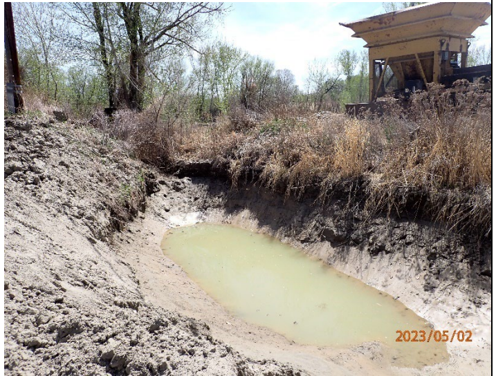
Photo #:14 Description: Facing east, photo of the truck wash water holding basin.
