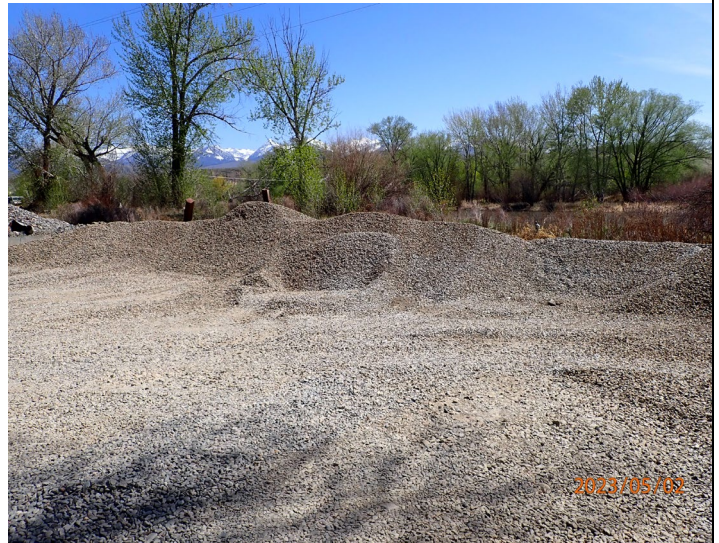
Photo #:12 Description: Facing east, photo of stockpile material for batch plant. .
