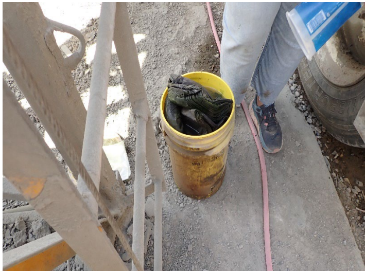
Photo #:15 Description: Facing down, photo of spill kit filled with water.
