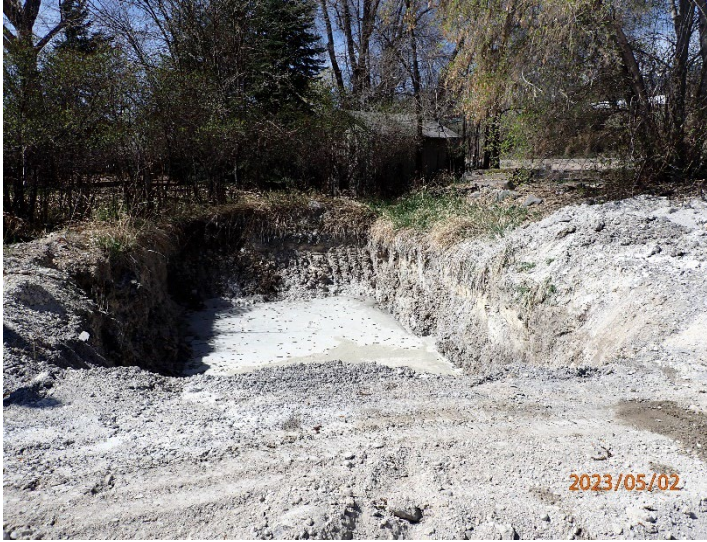
Photo #:09 Description: Facing south, photo of the truck washout area.
