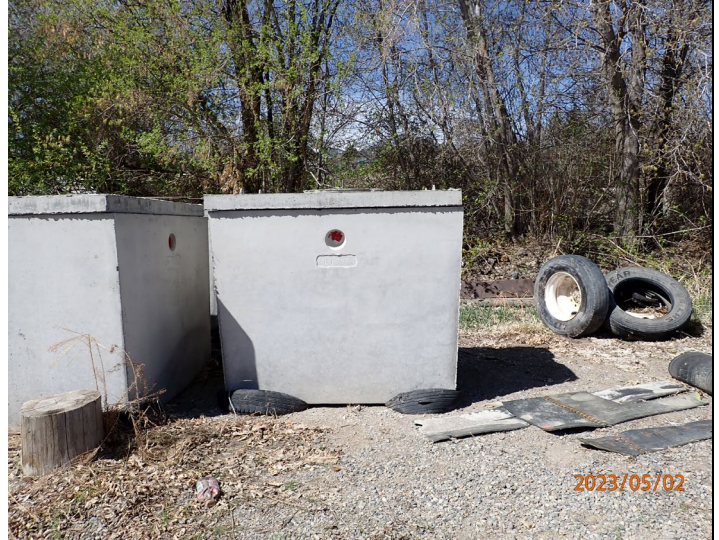
Photo #:06 Description: Facing west, photo of poured concrete septic tank.
