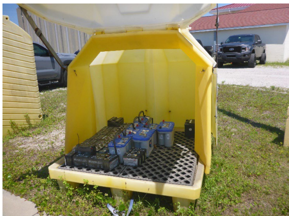
Photo 4: Universal waste batteries on a pallet that is equipped with a cover and lid.
