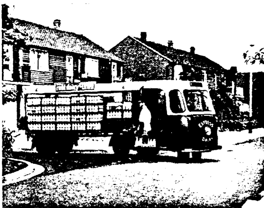
In London, an articulated vehicle, battery powered, carries 110 cases of pints, travels up to 32 miles per day on one charge. Express Dairy uses these for delivery to customers as well as to distribution points.
