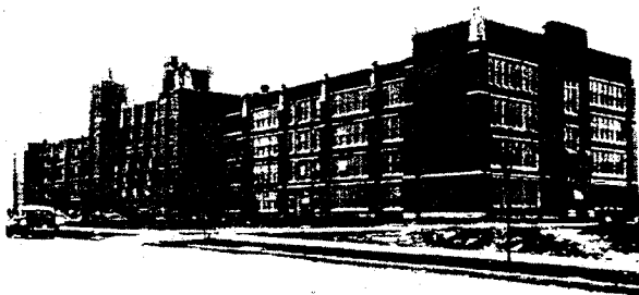
ADVERTISERS STUDIOS Mount Pleasant Regional Senior High School, Providence, R. I., where lead is used in the laboratory plumbing.
