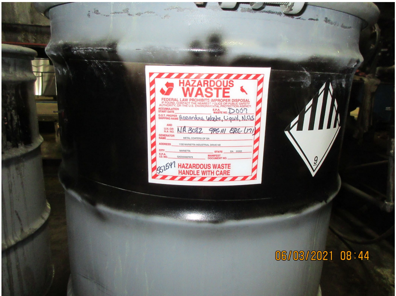
Photo 2 – Hazardous waste oil generated from oil skimming tank shown in Photo 1
