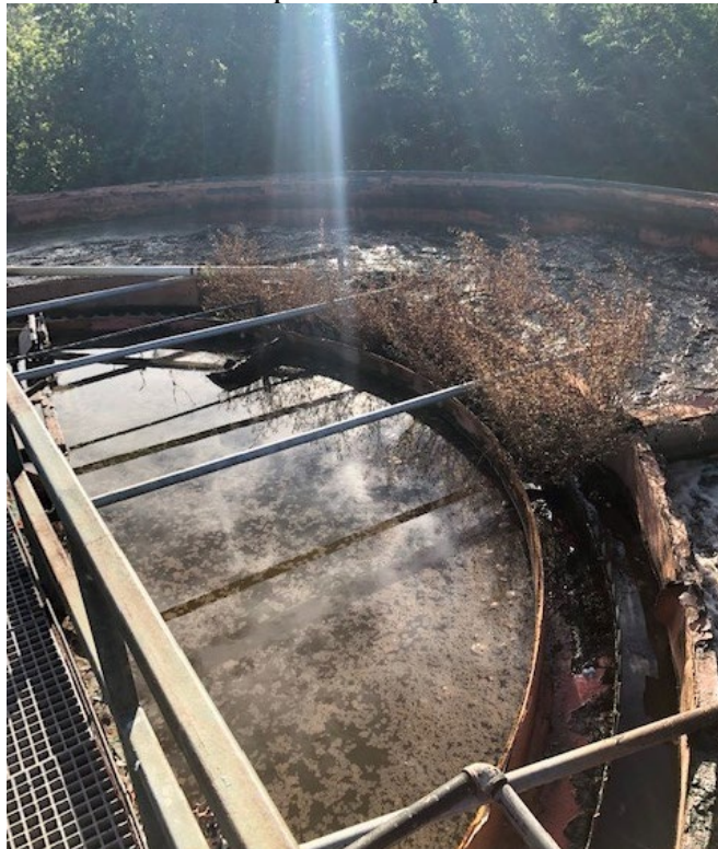
Photo #4: Vessup Plant Topside
