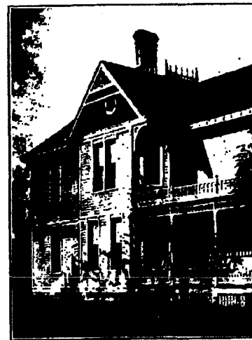
An S. W. P. Residence of J. E. Applegate, Rogers, Timmer, & Co., Sash.
