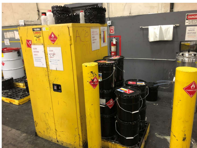
Photo 9: Solvent Recovery System 1.
