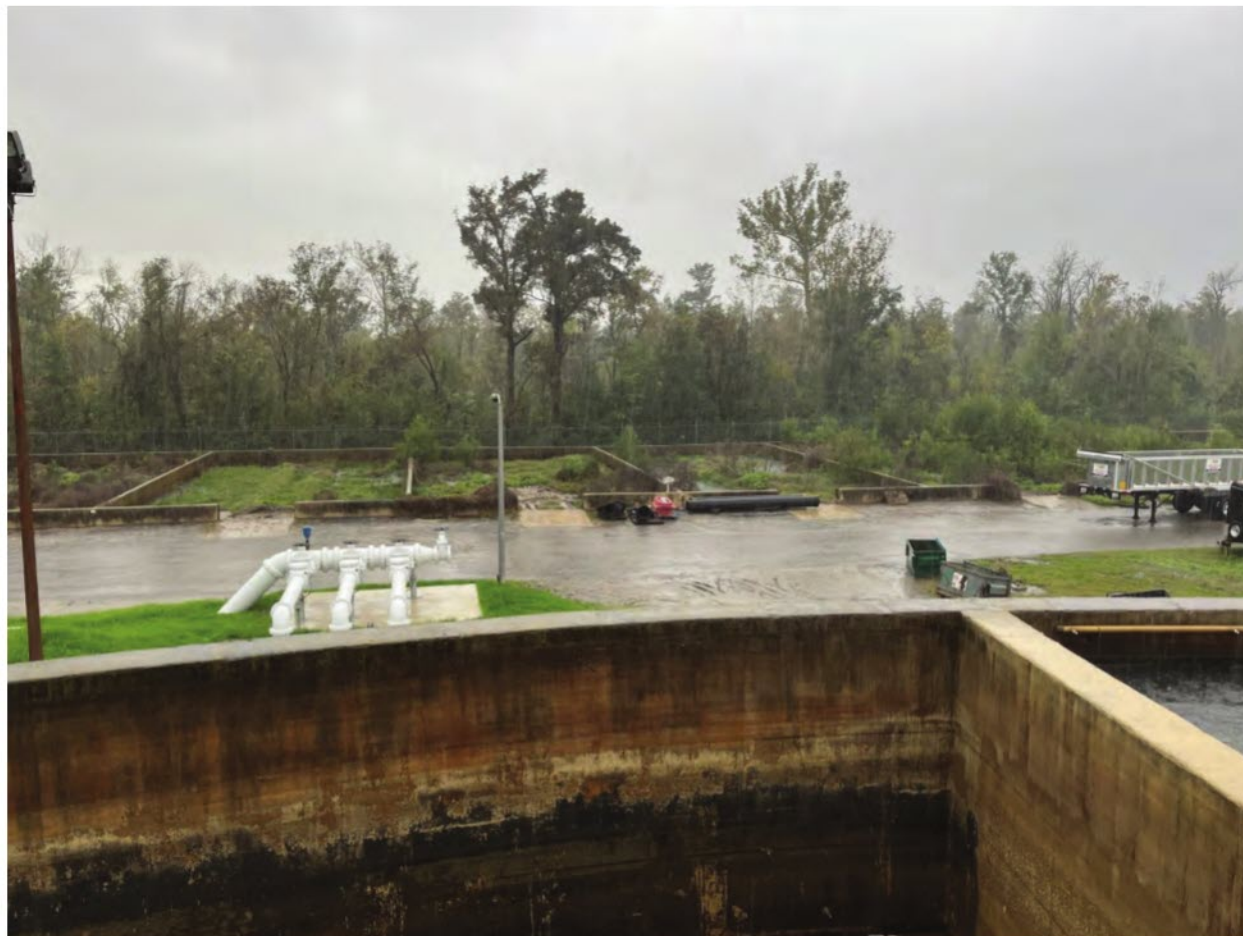
Woodland Treatment Overgrown Drying Beds
