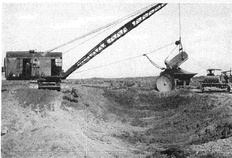
Above—Where the John Phillips Company built a 30-inch concrete siphon to carry a lateral under the main canal in a 38-foot cut
