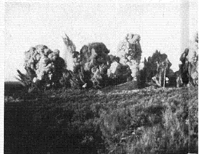
Twenty-eight and one-half tons of dynamite were set off in one day by Mittry Brothers to break up rock formations
