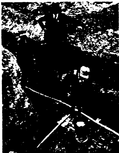
Joining lead pipe for service lines in Detroit housing project.
