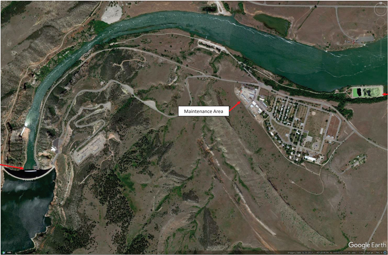
Yellowtail Dam and Maintenance Facility – Site Overview
