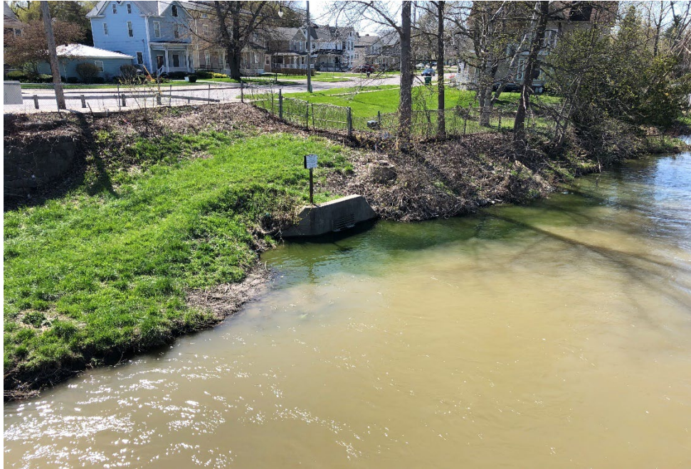
Photo #3. Algae were observed discharging from the City of Batavia WPCP outfall.
