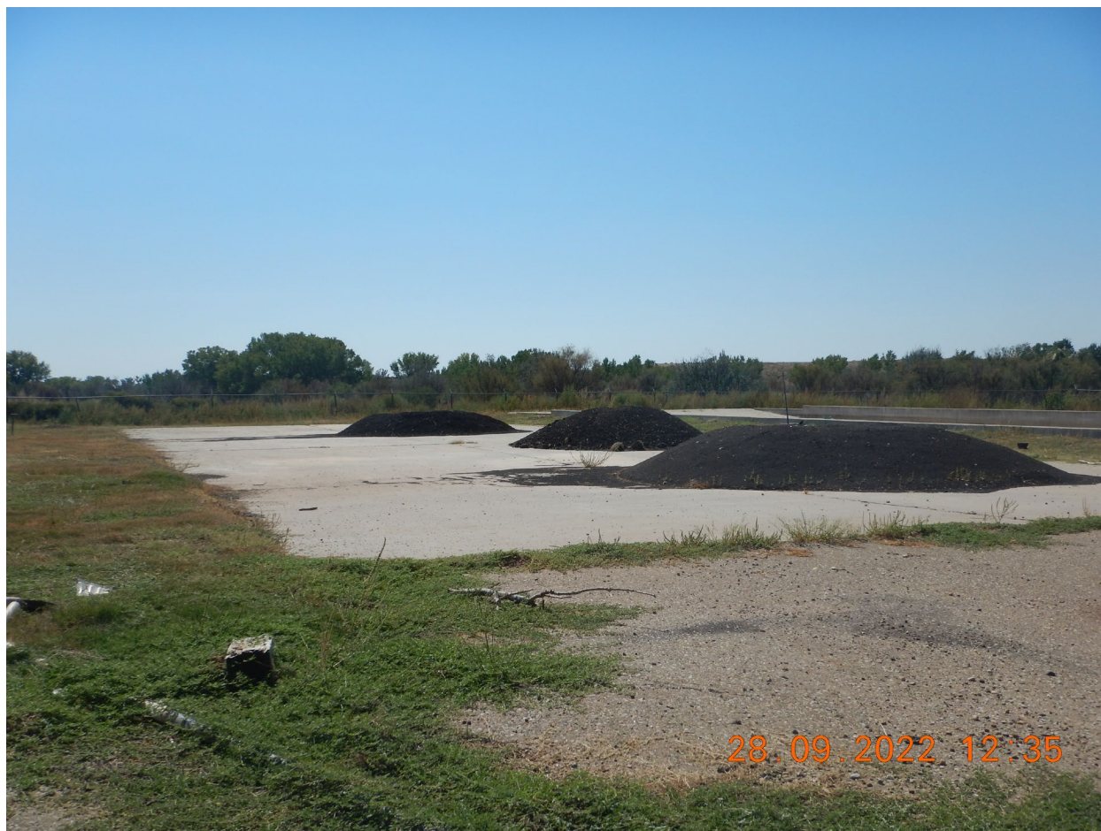
View of the three (3) staged sludge piles observed and awaiting transport and disposal. (DSCN2343). Photographed by D. Esparza
