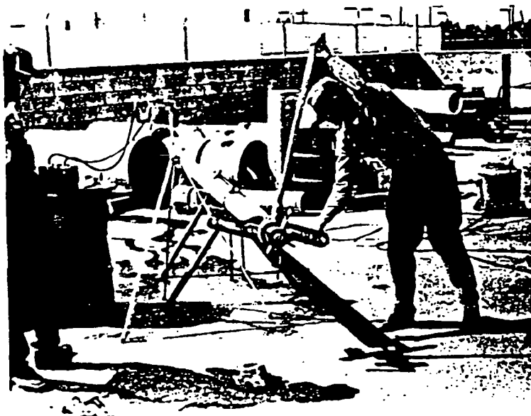
FIGURE 18. Use of manual lathe on 4-inch pressure pipe.
