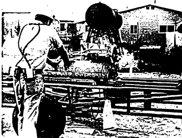
FIGURE 12. Doty tool, cutting.
