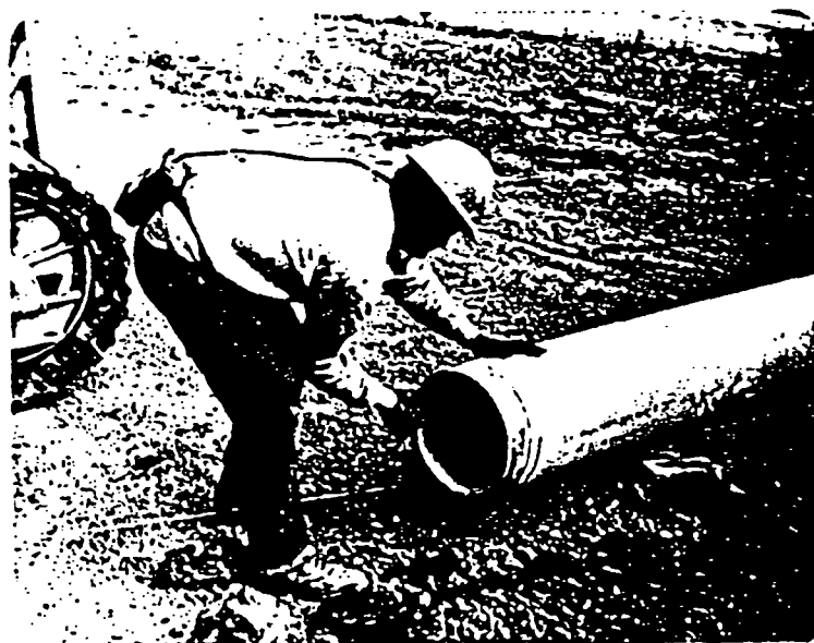
FIGURE 4. Lubricating pipe at trench.
