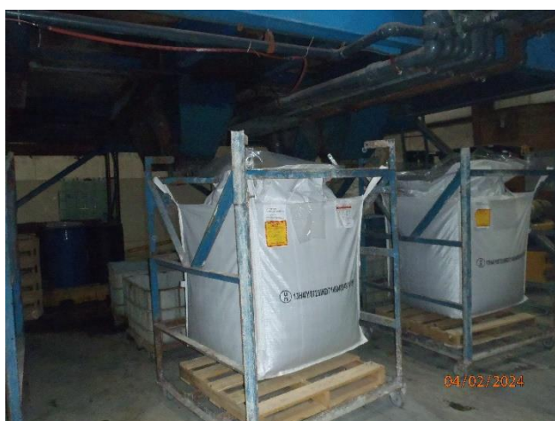
Picture 20 – WWTP CAA open supersacks
