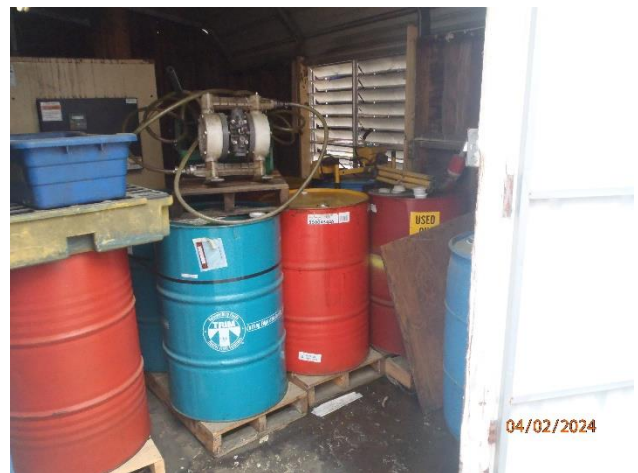
Picture 29 – Air Compressor Room used oil containers
