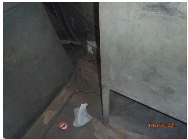
Picture 12 – Clean sand blast media released to ground
