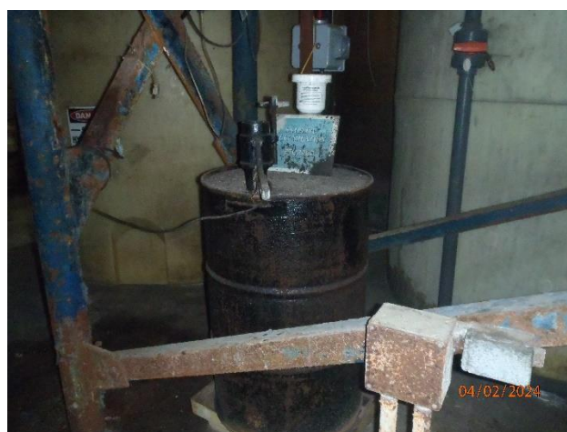
Picture 23 – WWTP aerosol can puncture SAA not labeled
