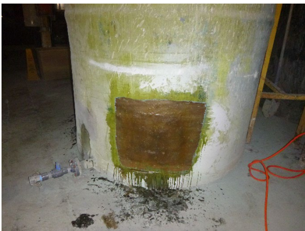
Photo 26: Tank WWT #2 (Tank 5).
