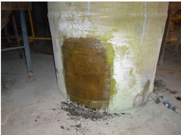
Photo 27: Tank WWT #2 (Tank 5).
