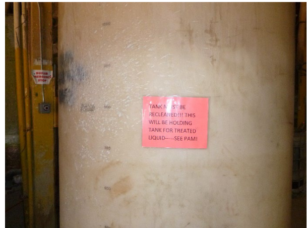
Photo 28: Tank WWT #3 (Tank 8).
