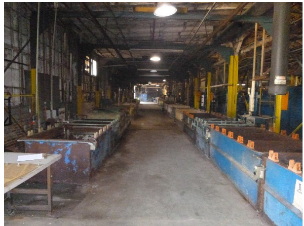
Photo 34: Aisle way in plant.
