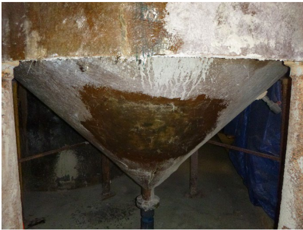
Photo 25: Tank WWT #1 (Tank 3).
